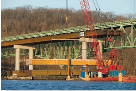
All photos: steel erection
